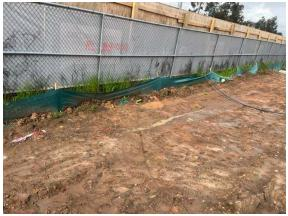
Photos 15 & 16: Sediment fence in place but to be maintained along the southern site boundary, Site 2
