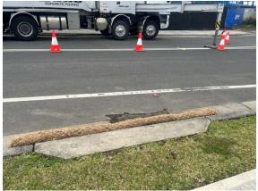
**Photo 18:** ERSED controls in place along Conferta Ave stormwater inlets
