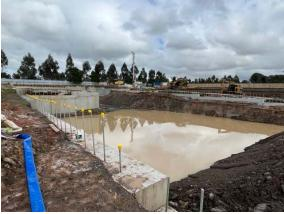
**Photo 8:** Water in basement excavation, Site 2. Capping beams installed.
